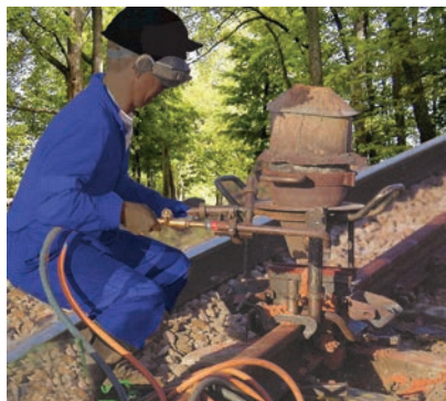
Figure 3.11 Thermit process for joining railway tracks
